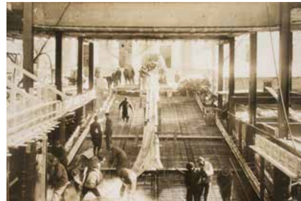
CCC workers built the DOI structure
